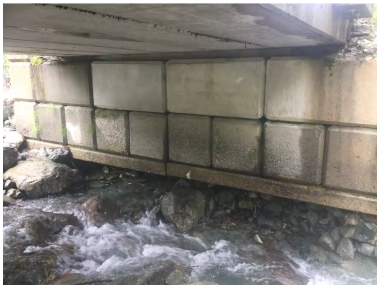
Left Bank Abutment when facing downstream
