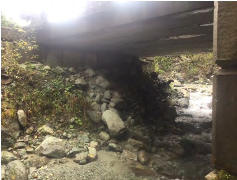
Right Bank Abutment when facing downstream
