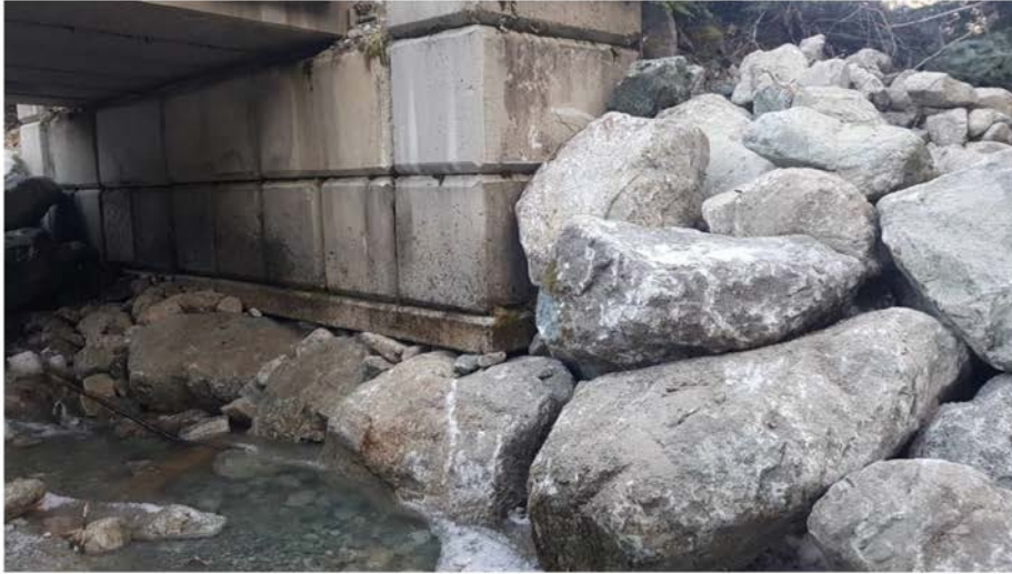
Town Abutment Upon Completion Of Repairs Looking Upstream – November 29 th , 2019
