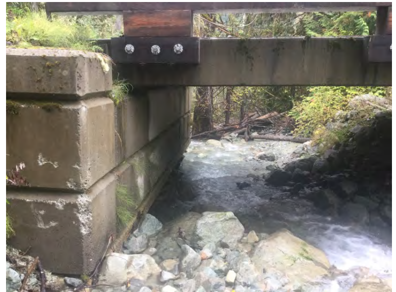
Left Bank Abutment when facing downstream
