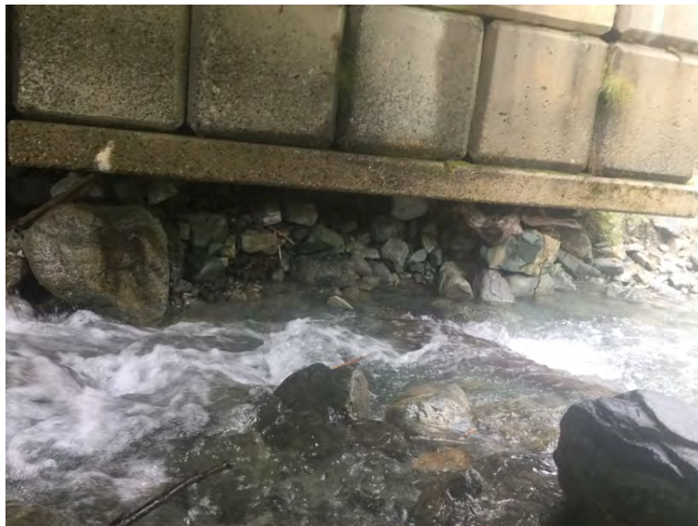
Left Bank Abutment when facing downstream
