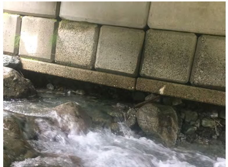
Left Bank Abutment when facing downstream
