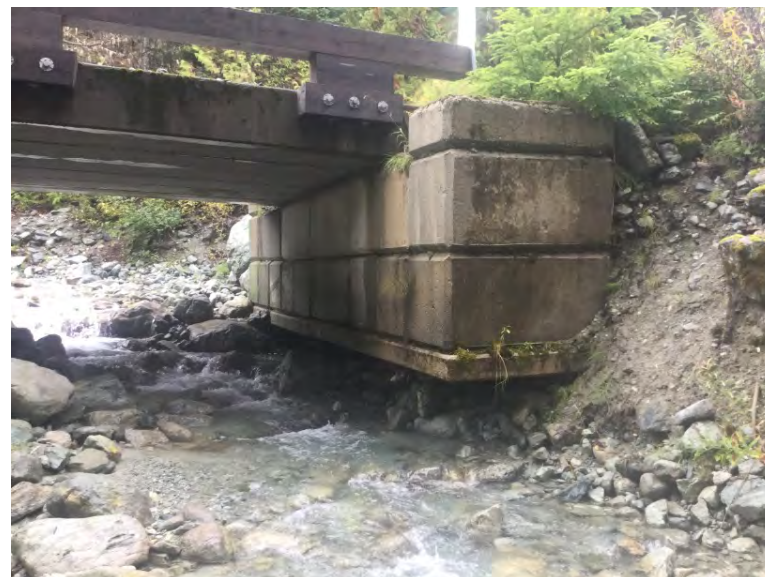
Left Bank Abutment when facing downstream
